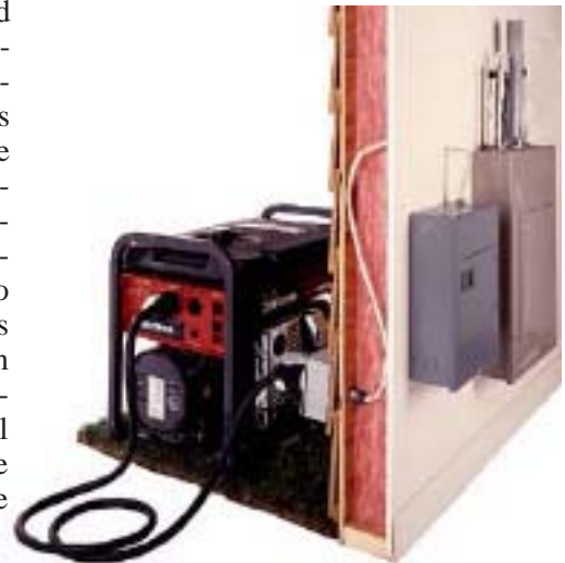
Typical Portable Generator Installation
