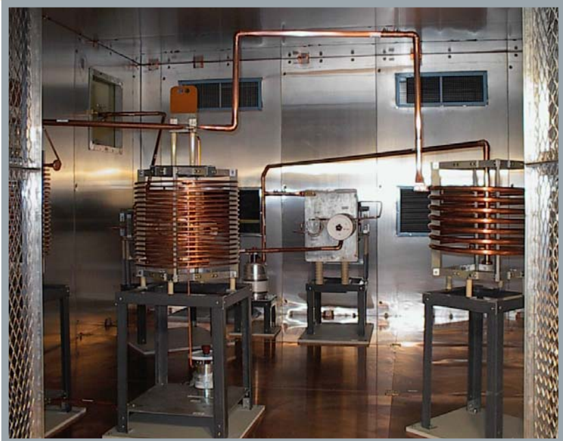
FIGURE 1: High Power MW Antenna Tuning Unit
